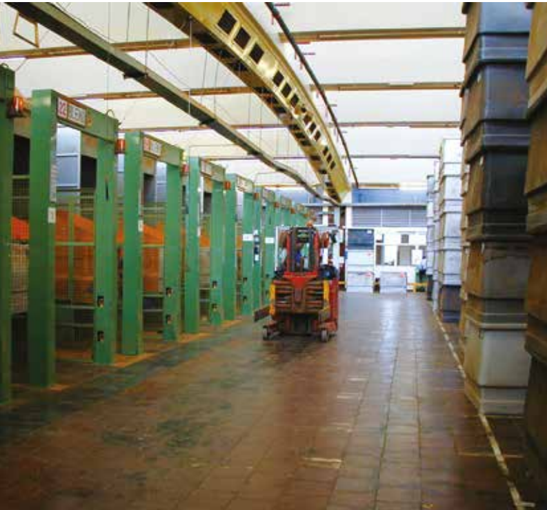
Automatic bin filling and delivery area within Cigarette Primary
