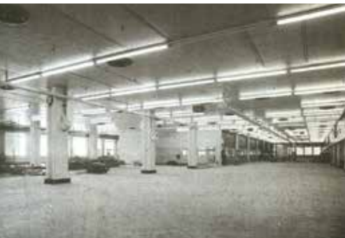
Construction on the third floor at Henry Street, which would become the new home for roll and bar production
