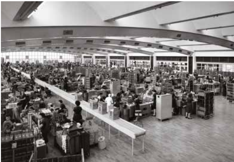
Packing: a wide view of the packing floor
